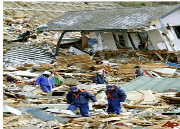
Figure 69. March 18: Firefighters and rescuers continue search operation in Onagawa, northern Japan. (AP Photo/Kyodo News)
