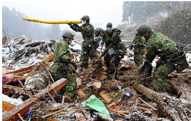
Figure 53. March 16: Rescue workers from Japan's Self-Defense Forces dig through the debris of houses that were destroyed in Minamisanriku, in Miyagi prefecture. Source: www.time.com
