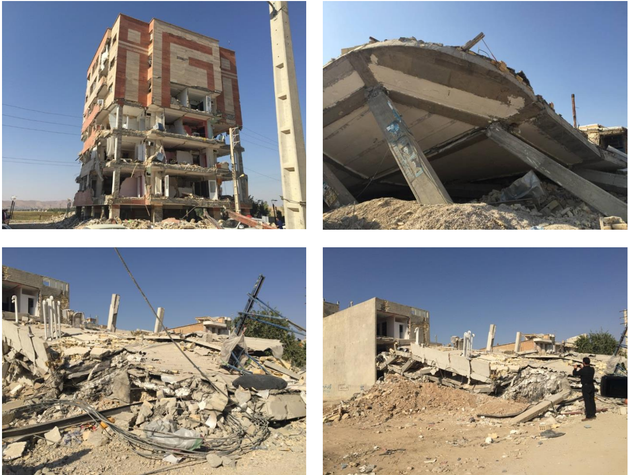
Fig 6. Collapsed buildings in Sarpol-e Zahab city
